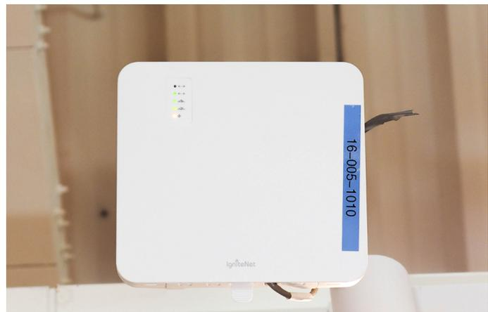
Figure 2 &3: APs are installed on the ceiling of the store to provide customers and store equipment with stable and high-performance Internet connection services
