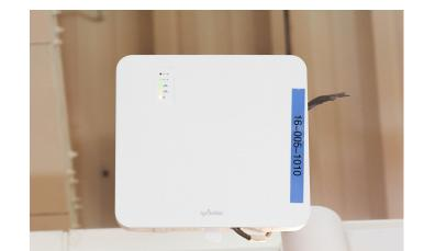
Figure 2 &3: APs are installed on the ceiling of the store to provide customers and store equipment with stable and high-performance Internet connection services
